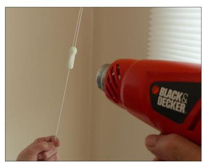
7. I have used a match or lighter to heat up tubing of this type when applied to wiring, but for this job I needed gentler heating to avoid damaging the connector or the cords. So I used an inexpensive Black & Decker 1375-watt heat gun to shrink the tubing around the connector.
